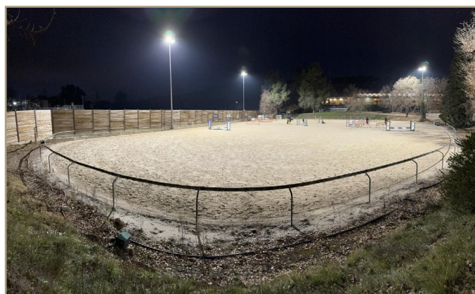
7 projectors in total for the 4 x 15 m high masts already in place.
