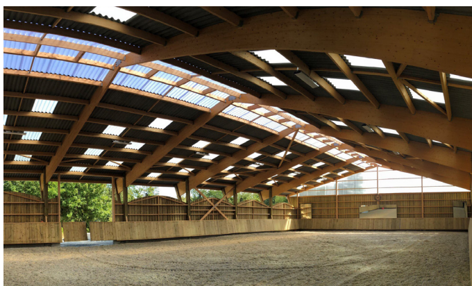
Glulam construction by James Charpente.
