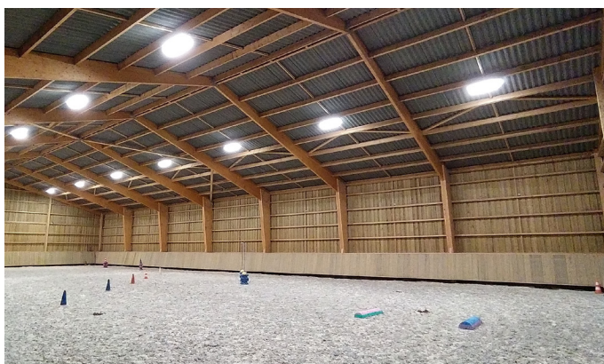
Glulam construction by James Charpente.
