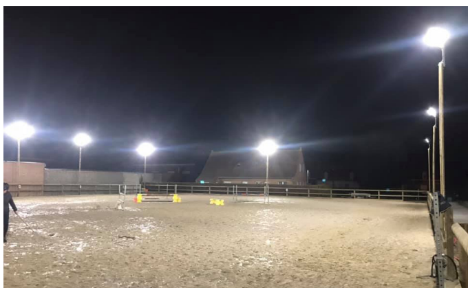
Lighting quality and uniformity (10 fixtures - 10 masts)
