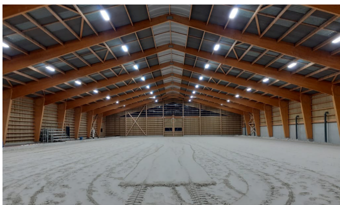
Quality of lighting on the ground (40 lighted luminaires for competition mode).
