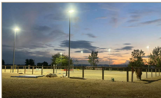
8 masts (8 m high) 8 fixtures PROXI-OUTDOOR-ARENA.
