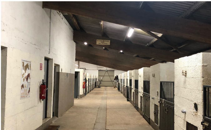
Optimized lighting within the driveways
